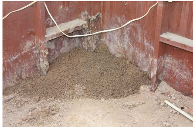
Photo 2: This second pile of dirt showed up overnight.
