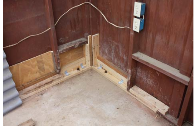
Photo 4: Since these patches were applied, Mr. Mole has not brought any more dirt into Mole Manor.
